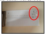
All lights can be turned off or on using the buttons on the right side of the control panel (Please DO NOT use the left *zone* buttons) these are for dimming and the lights are not dimmable. (if these controls are used the lights will flicker).
